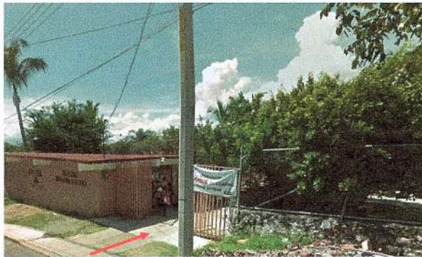
F1: Fachada principal E.E.S. Mazatepec
