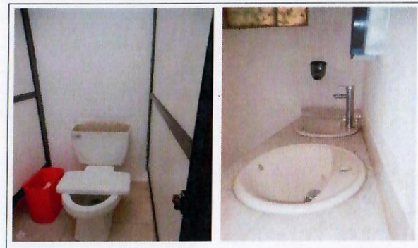
F11: Sanitarios a rehabilitar
